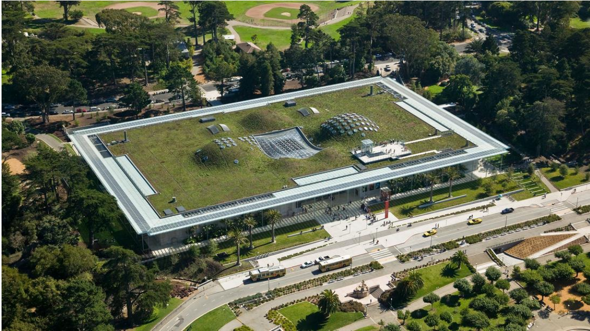
Figure 27: California Academy of Sciences, the green roof houses local plants and solar panels to reduce the energy consumption and prevent heat absorption. (Weston, 2011, 196) https://s3.amazonaws.com/swacdn/wp-content/uploads/2015/09/18074214/73fb0cbc_californiaacademyofsciences-7031_1100x1100-1100x619.jpg
