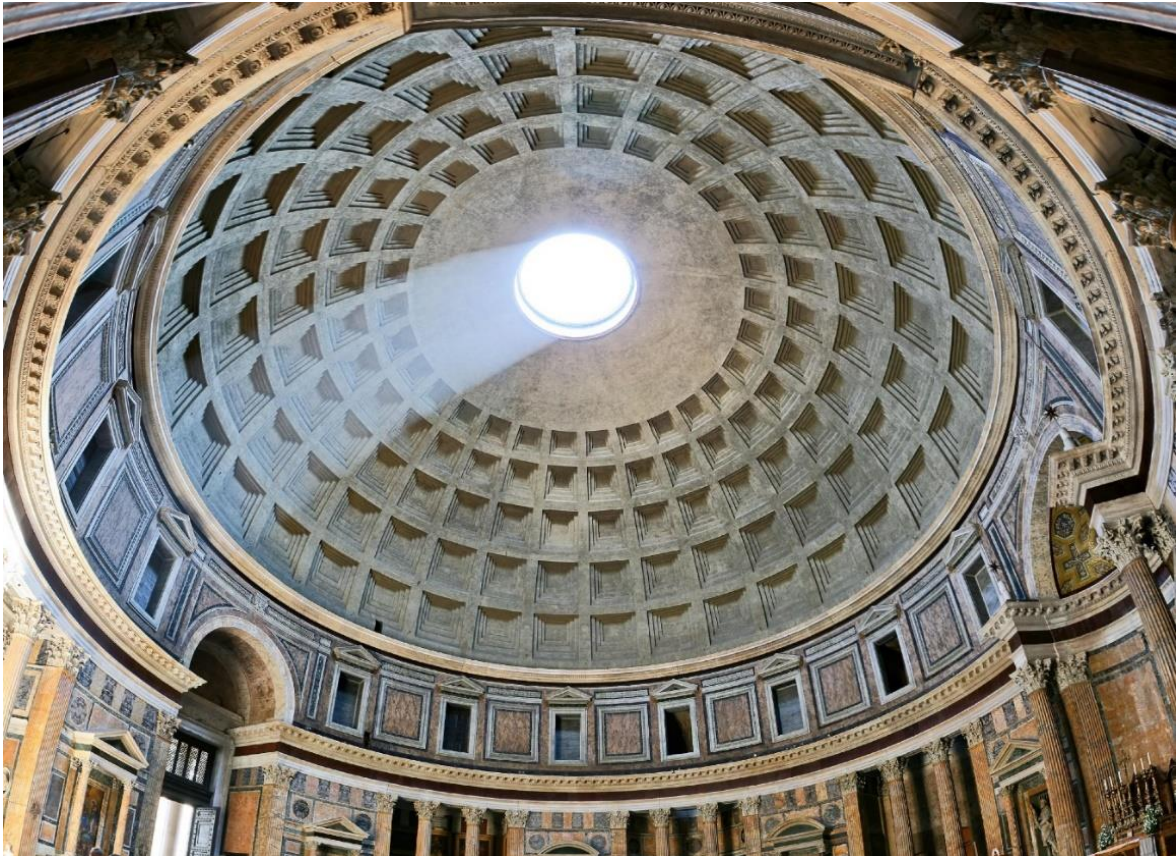
Figure 2: The Rotunda with the opening at the top. The squares and circles form a total symmetry, and the oculus allows light to enter the building.
