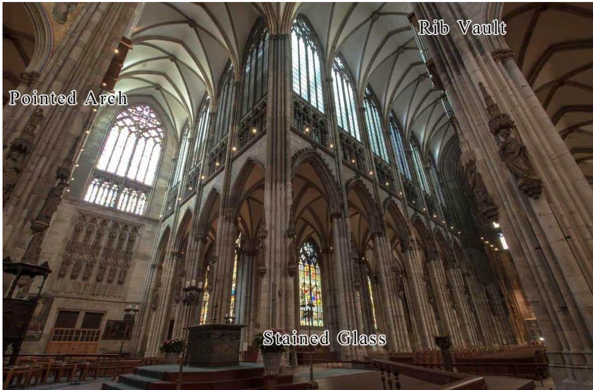
Figure 5: Interior view of the Cologne Cathedral. The pointed arches, the rib vault, and the stained glass can be seen. Additional texts written by the author.
