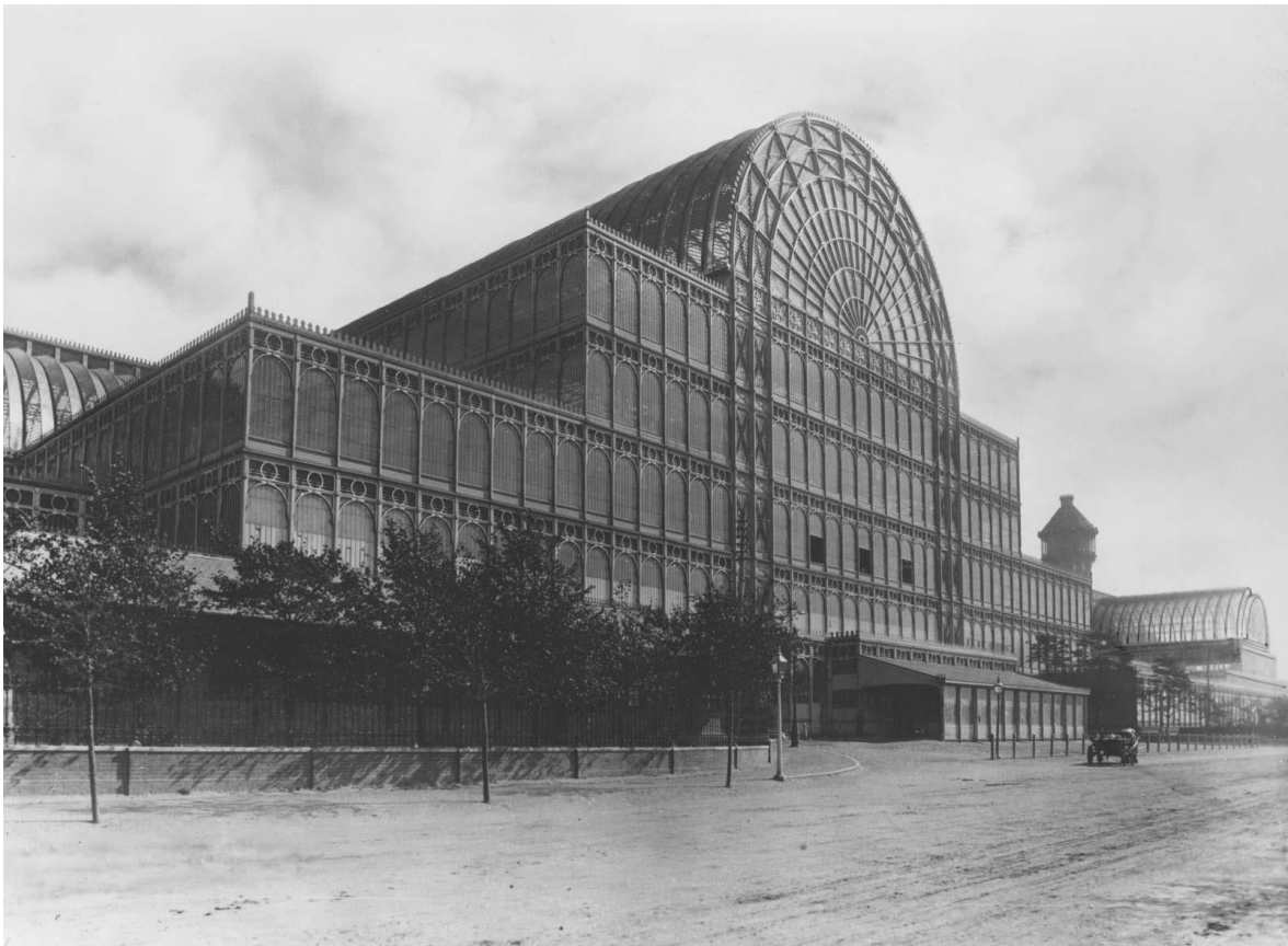
Figure 15: The Crystal Palace in Hyde Park by Joseph Paxton, a glass/ metal construction built in 1851 to house the Great Exhibition of the Works of All Nations (Pile, 2009, p.246). https://www.britannica.com/topic/Crystal-Palace-building-London
