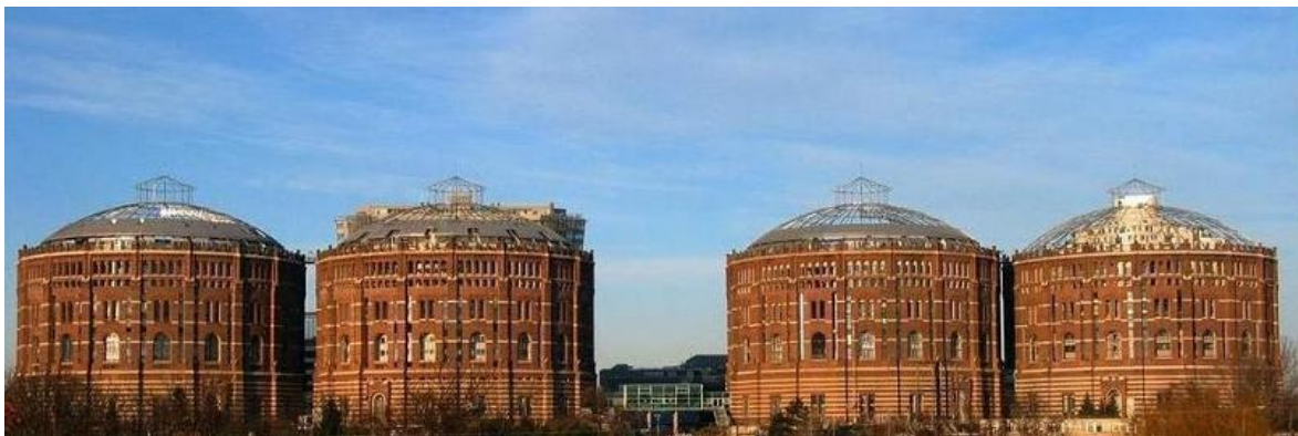
Figure 24: Southside view of the Vienna gasometers.
