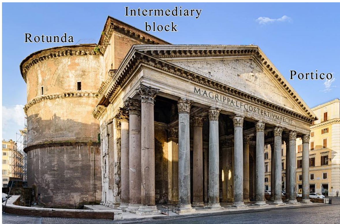
Figure 1: Exterior view of the Pantheon and its three structural elements, additional texts written by the author.
