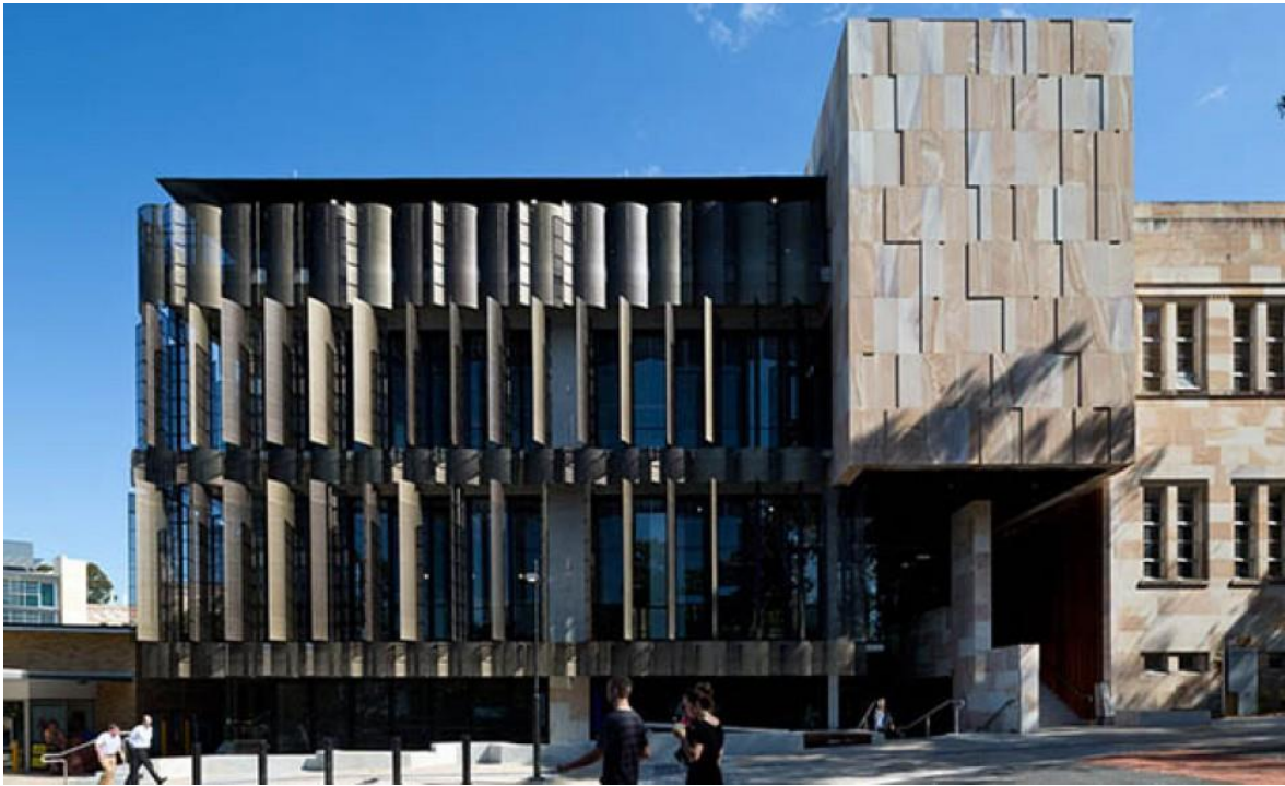
Figure 2.4. First public structure built with structural Geopolymer Concrete: The University of Queensland, Australia, 2014
