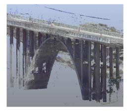
Figure 2: The texture-mapped point cloud of the Çayırhan Bridge.
