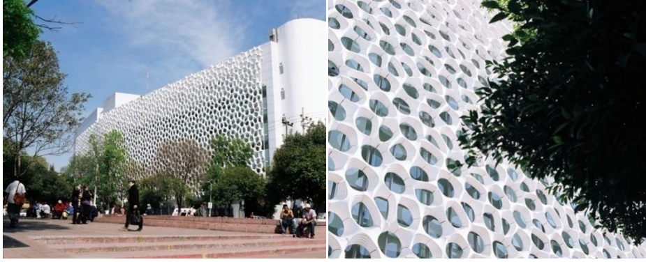
Resim 87. Manuel Gea Gonzalez Hastanesi, Duman Yiyen Akıllı Malzeme Cephe Sistemi, Elegant Embellishments Tasarım, Mexico City, 2013(URL-60).
