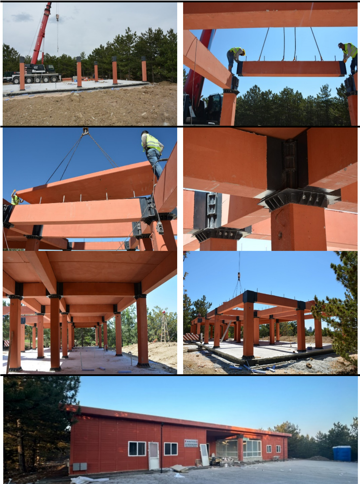
Fig. 1.5. Completely demountable housing construction with CDW-based geopolymer concrete
