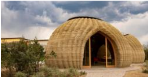
3D Printed TECLA Habitat Project (Massa Lombarda, Italy)
