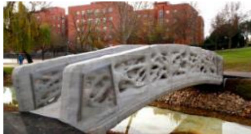
Castilla La Mancha Bridge Printed in 3D (Madrid, Spain)
