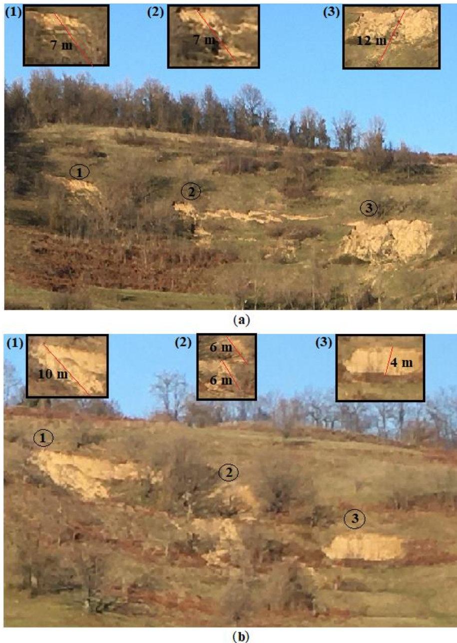
Figure 4.7. Some typical triggered shallow landslides view in the study area: (a-b) after November 2023 rainfall from field photographs.
