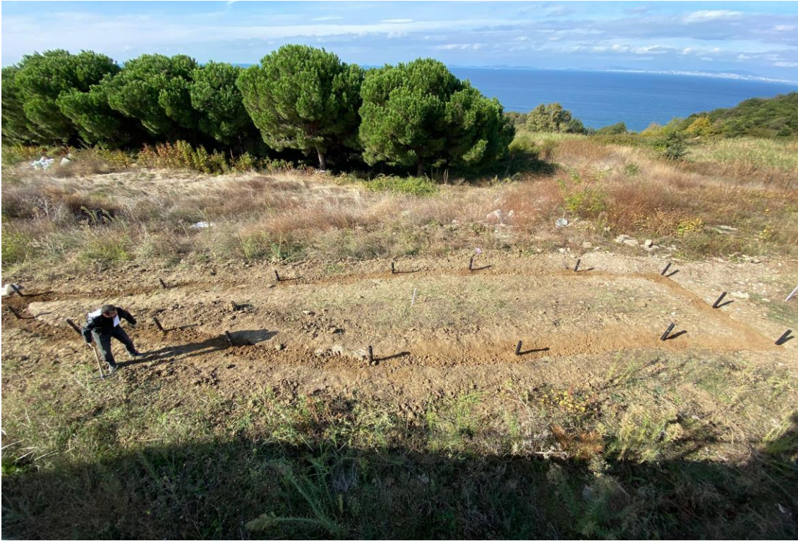
Figure 42. The completion of the entire fiber cable channel area before monitoring
