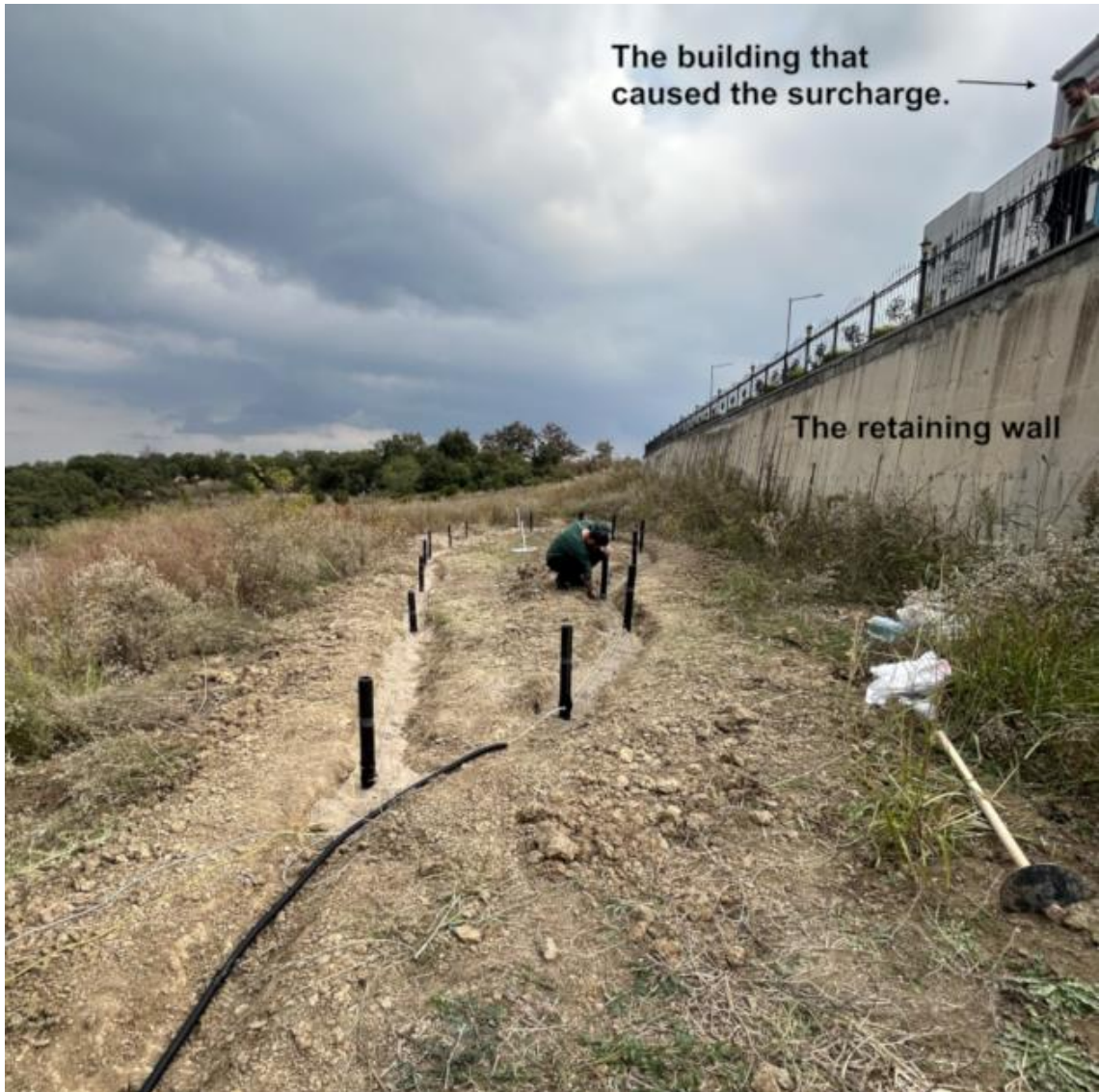
Figure 25. The retaining wall and building adjacent to the monitoring area
