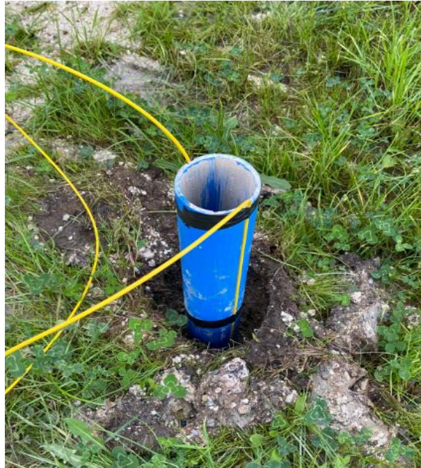
Figure 16. Inclinometer pipe and fiber cables in the hole drilled with a hand auger
