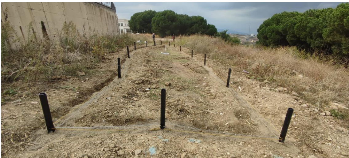
Figure 39. The entire configuration, after cushioning with sand
