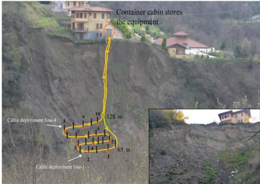
Figure 4. Fiber Optic Cable configuration at the landslide site in Bahçecik, Kocaeli (Arslan Kelam et al., 2022)
