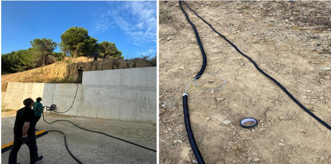
Figure 43. Fiber protection inclinometer pipes
