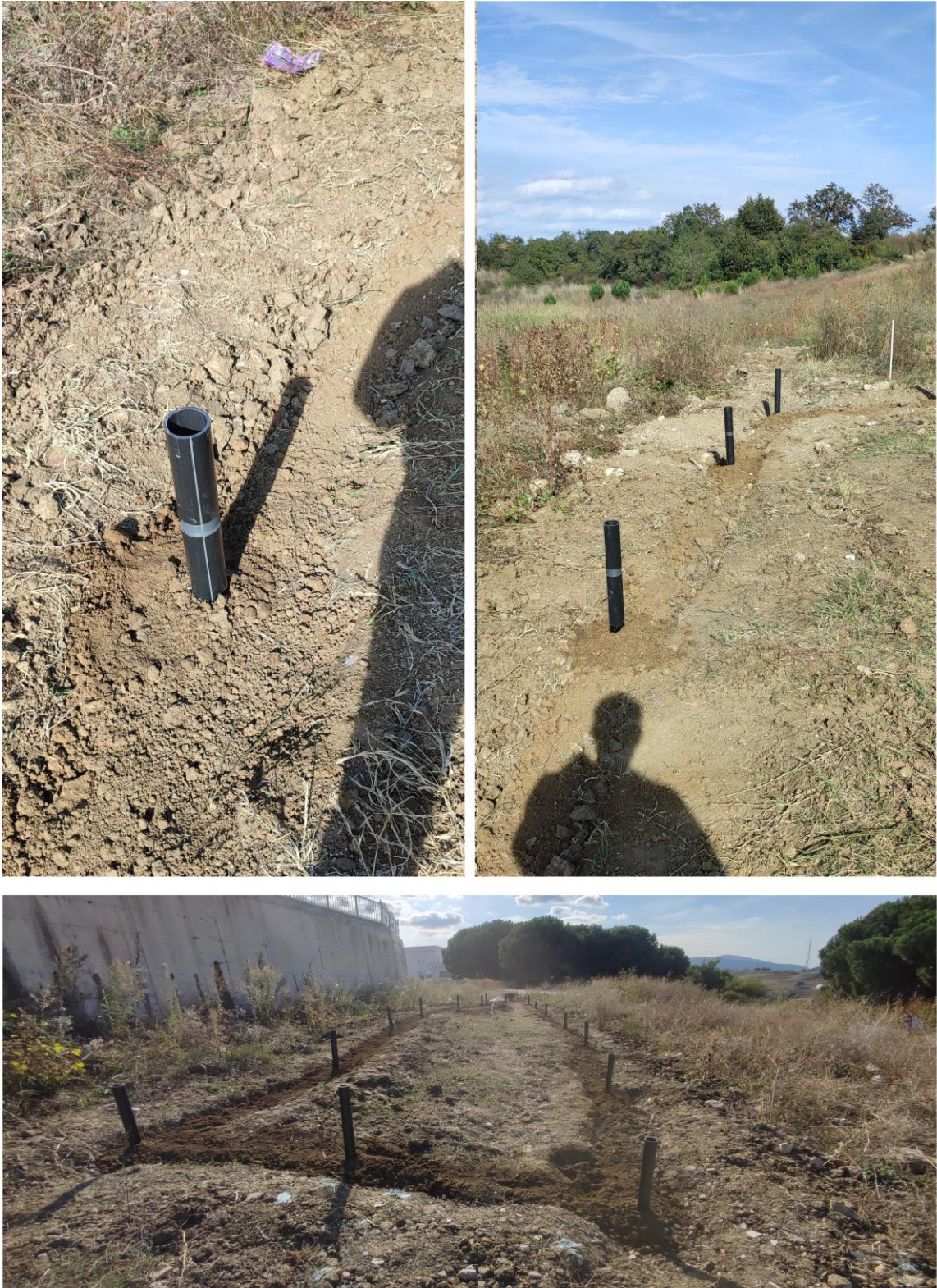
Figure 41. The completion of the entire fiber cable channel area
