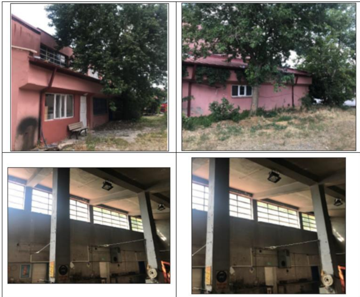
Figure 6.7. Photographs of Building #4
