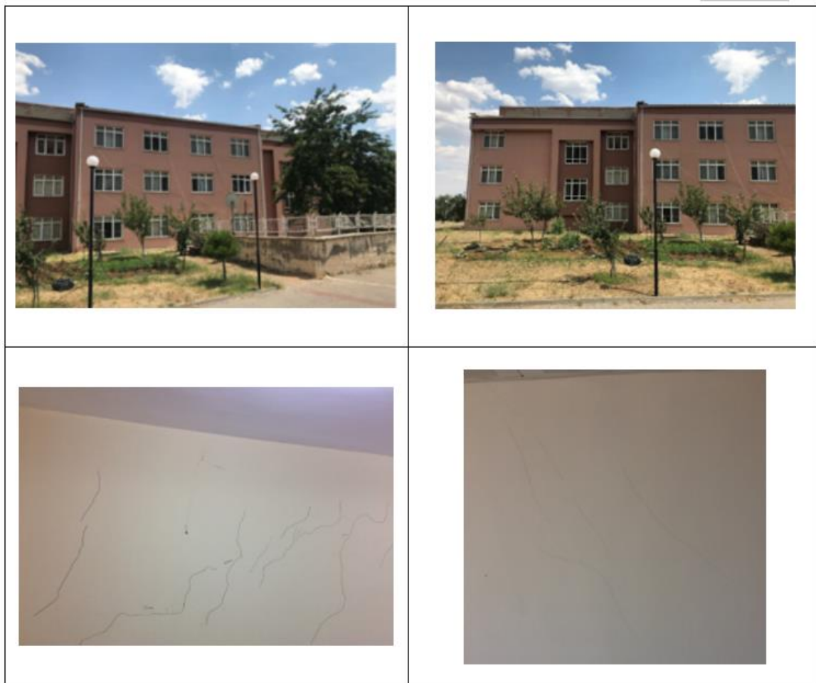
Figure 6.11. Photographs of Building #6
