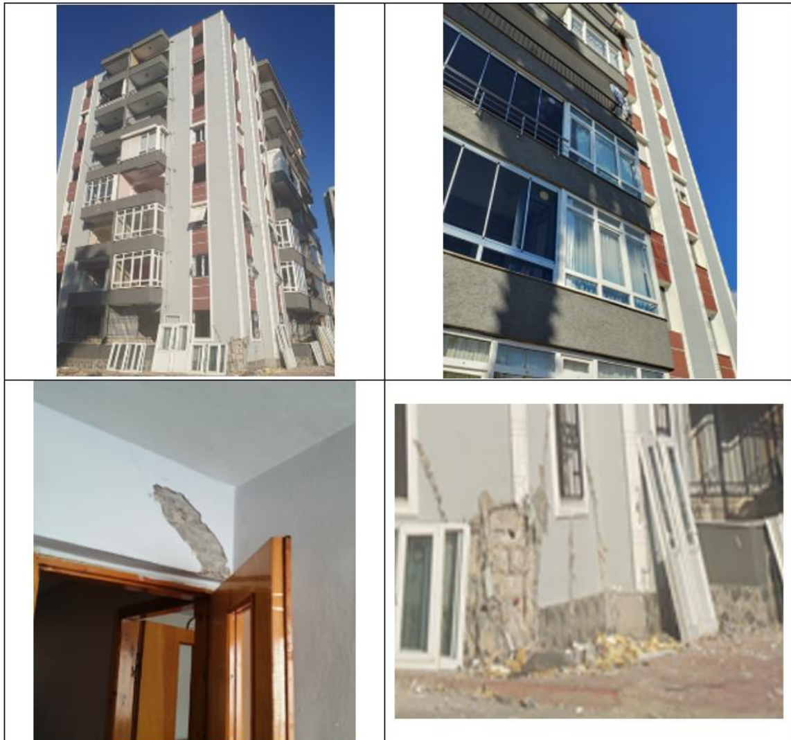
Figure 6.13. Photographs of Building #7
