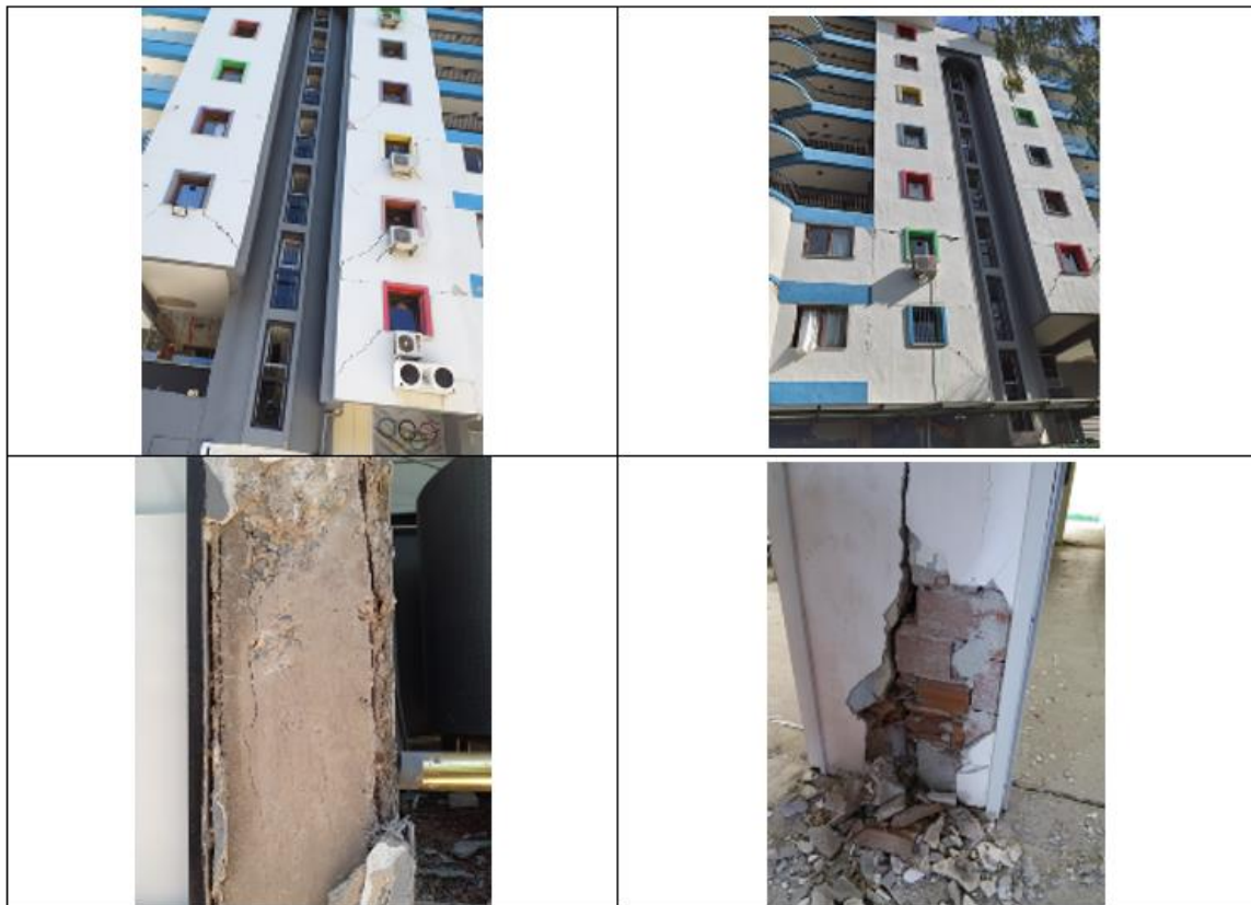
Figure 6.25. Photographs of Building #13
