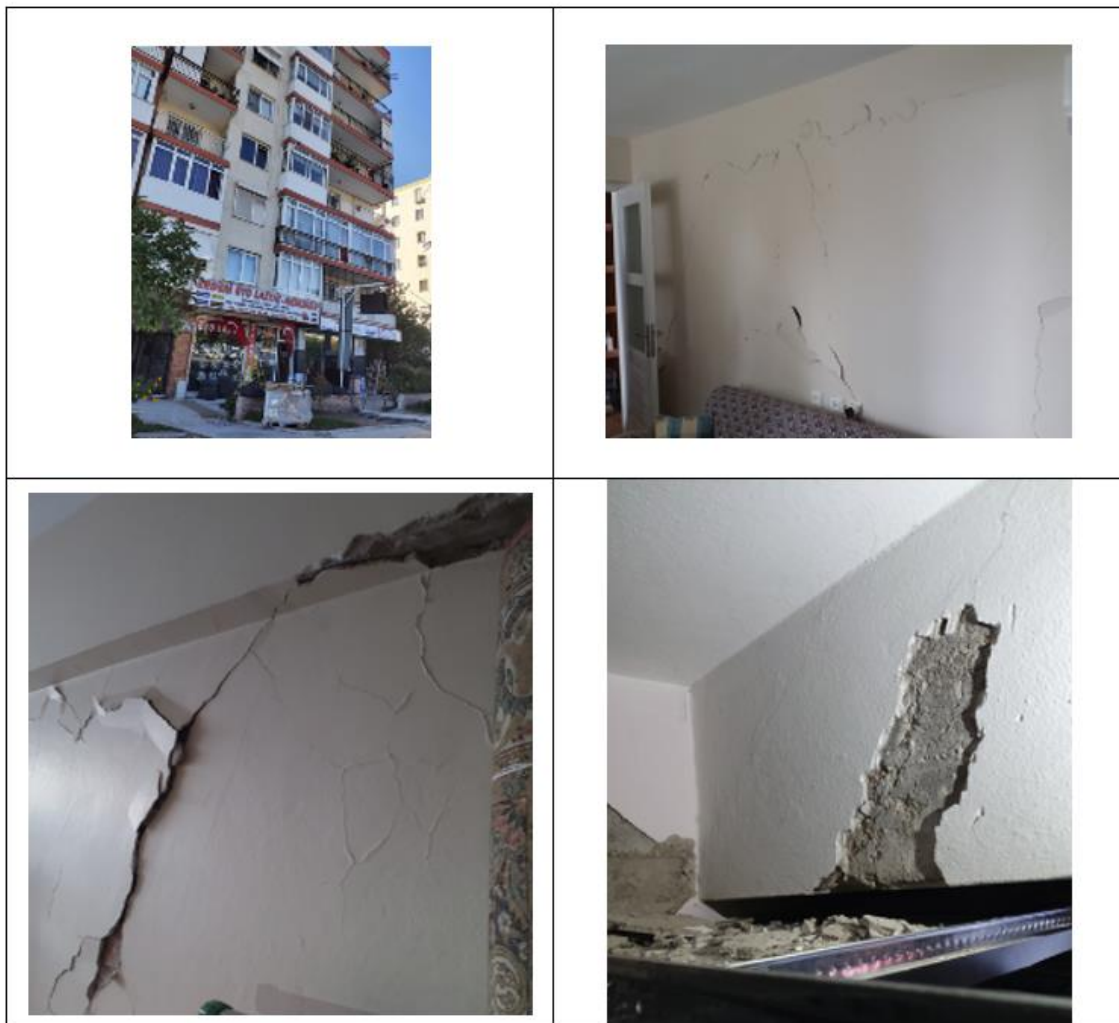
Figure 6.17. Photographs of Building #9
