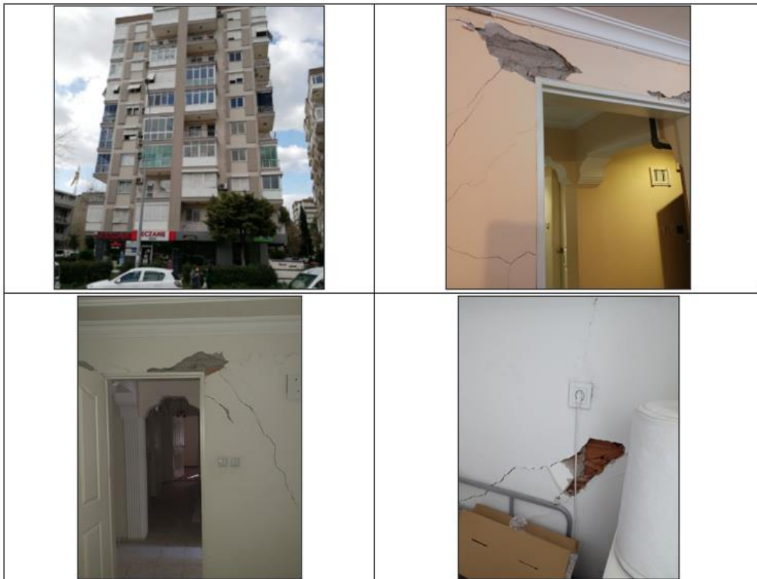
Figure 6.29. Photographs of Building #15
