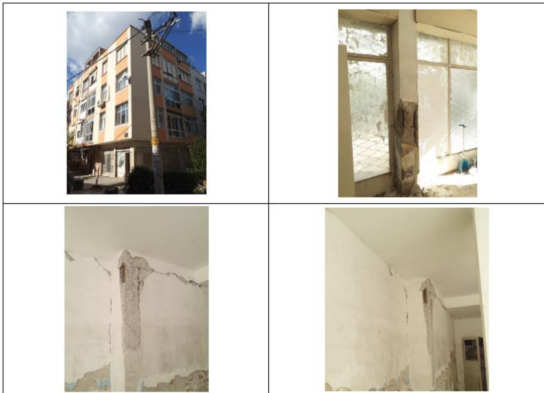
Figure 6.21. Photographs of Building #11
