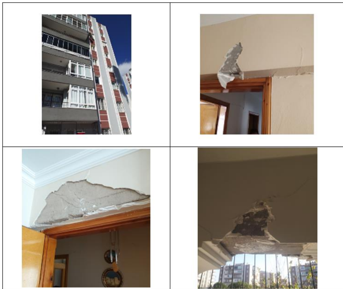
Figure 6.15. Photographs of Building #8
