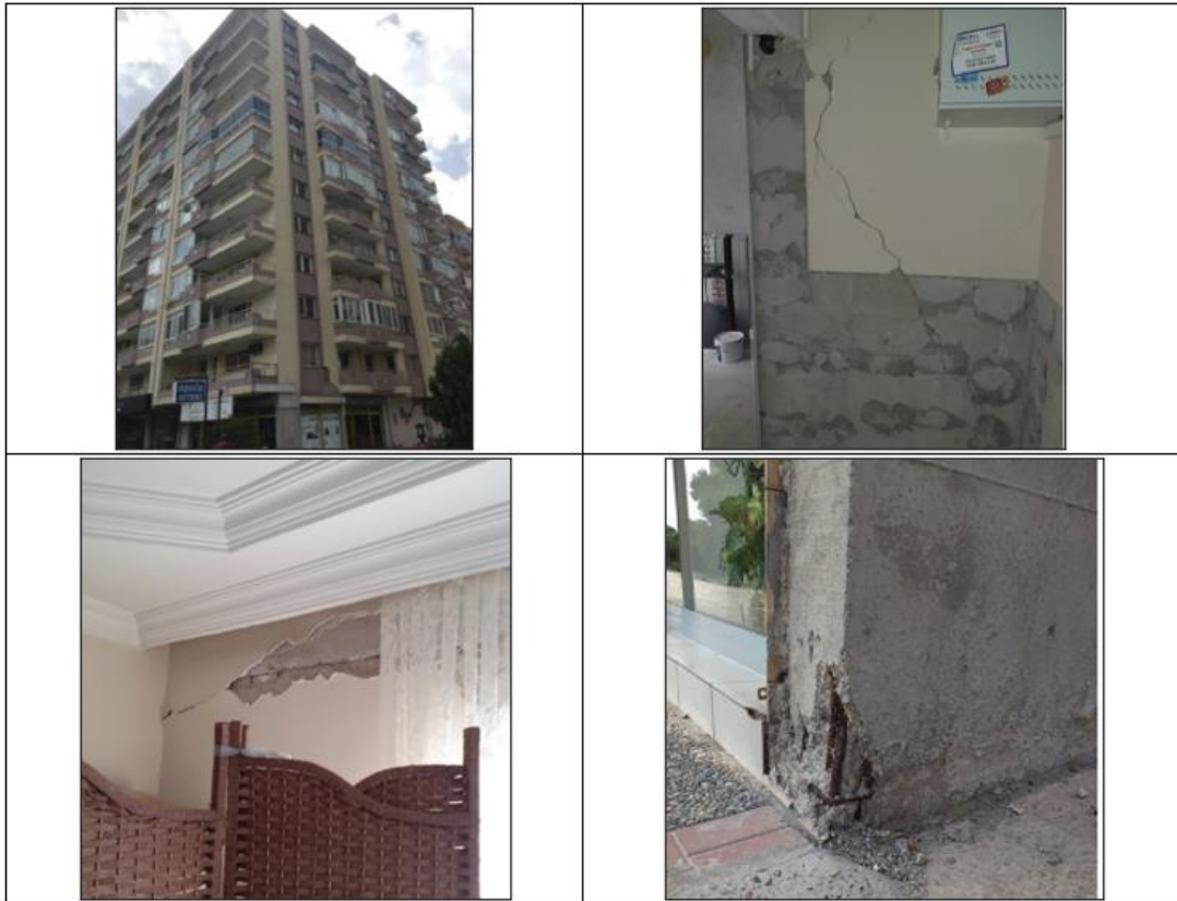
Figure 6.27. Photographs of Building #14
