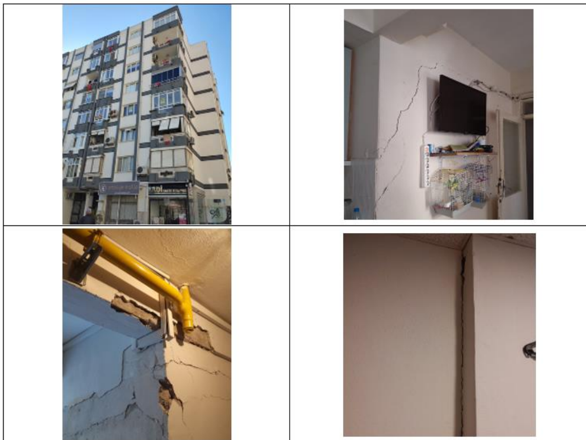
Figure 6.23. Photographs of Building #12
