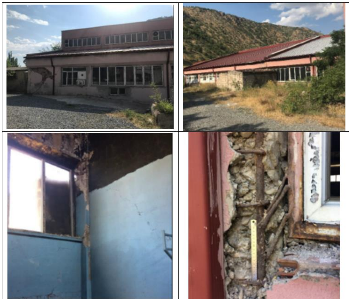
Figure 6.9. Photographs of Building #5
