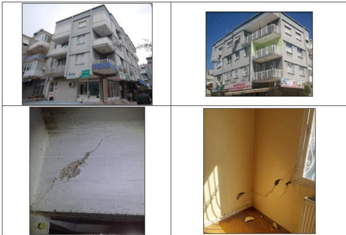
Figure 6.19. Photographs of Building #10
