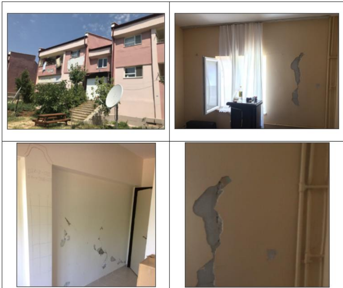
Figure 6.3. Photographs of Building #2
