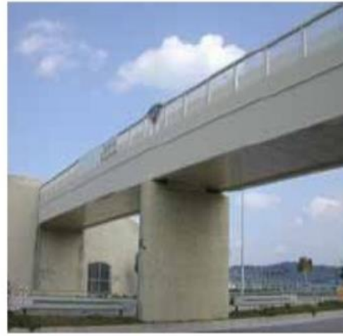
Figure 2.4 A pedestrian bridge in Okinawa Japan made of hybrid composite structure [13].
