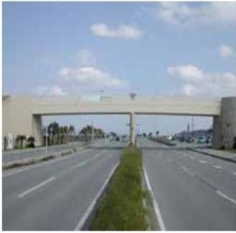
Figure 2.4 A pedestrian bridge in Okinawa Japan made of hybrid composite structure [13].
