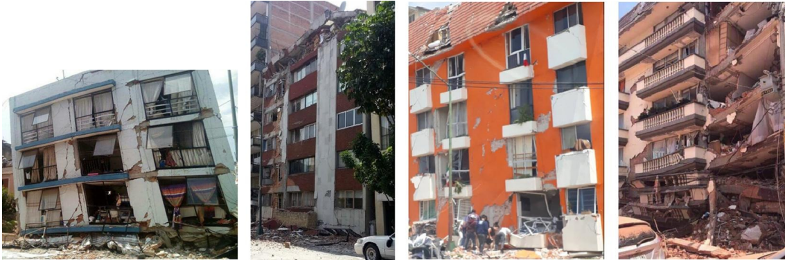
Figure 2.4 Formation of a Soft Story Mechanism After Mexico City 2007 Earthquake[21]
