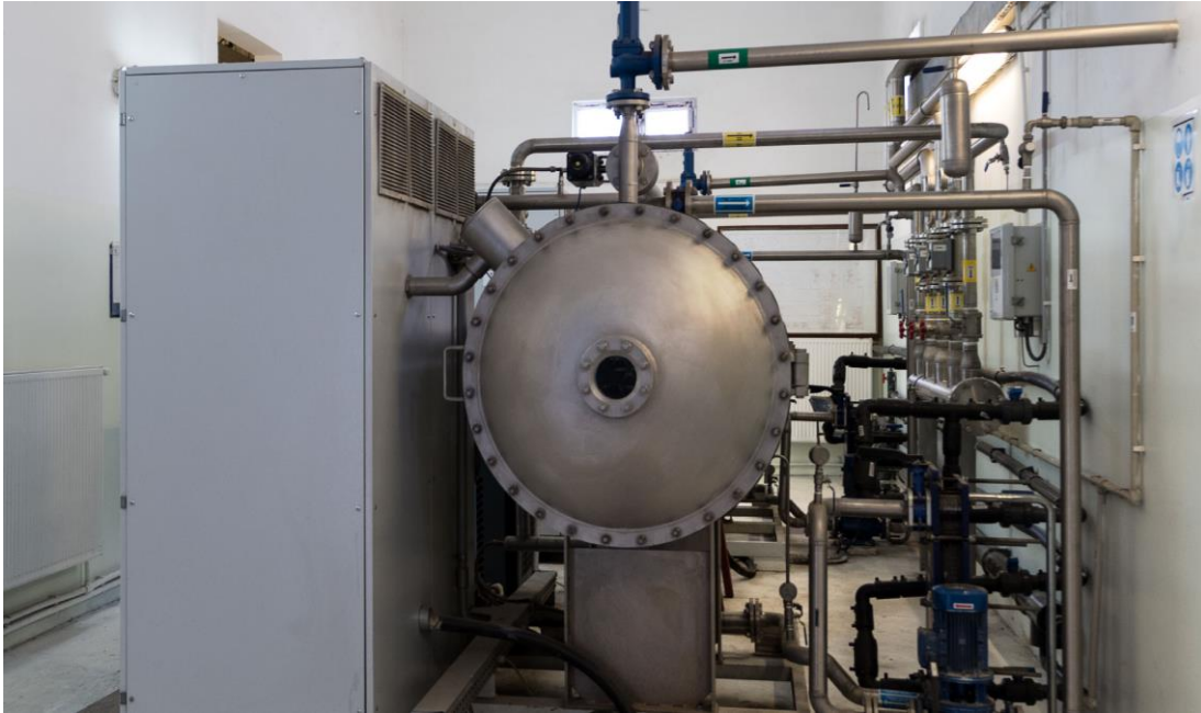
Figure 2.2.2.1 Ozone Disinfection System
