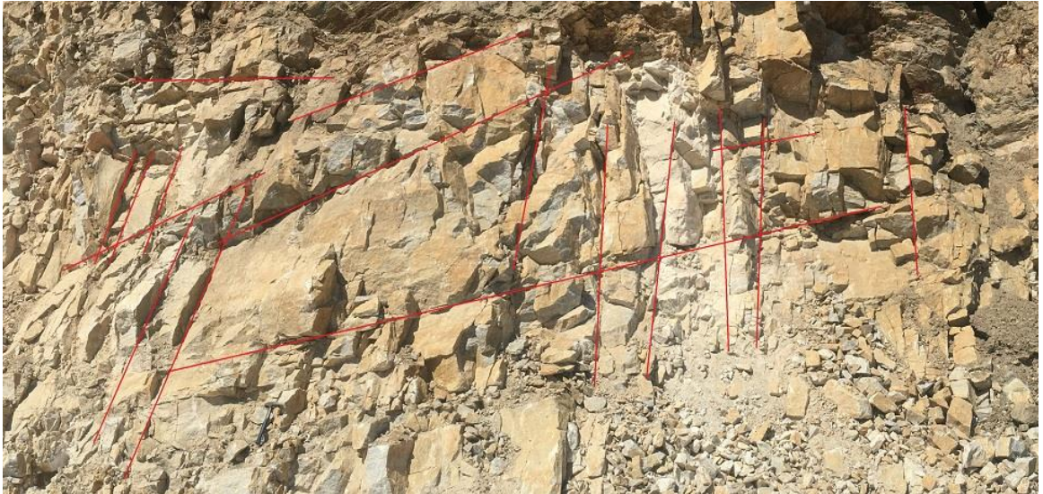
Figure 22. The general appearance of the rock mass in the first quarry
