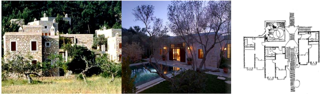
Şekil ( 126,127,128 ) Demir Tatil Köyü, Bodrum, Türkiye, Demir Holiday Village, Recipient of the Aga Khan Award for Architecture , The Aga Khan Award for Architecture, www.akdn.org, 1992
