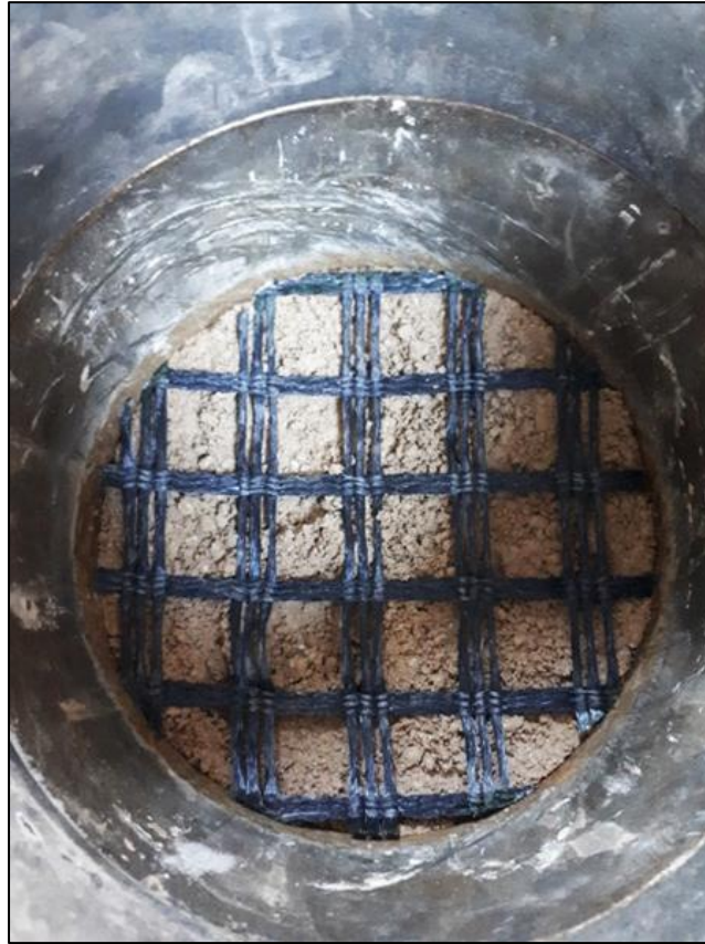
Figure 3.19 A geogrid placed between compacted soil layers.
