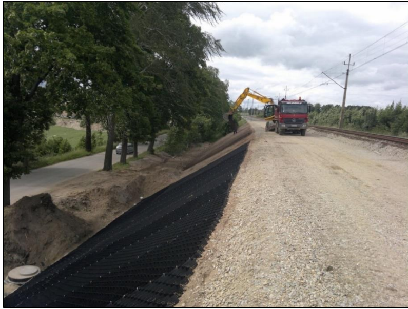
Figure 2.1 A road embankment reinforced with geosynthetic.
