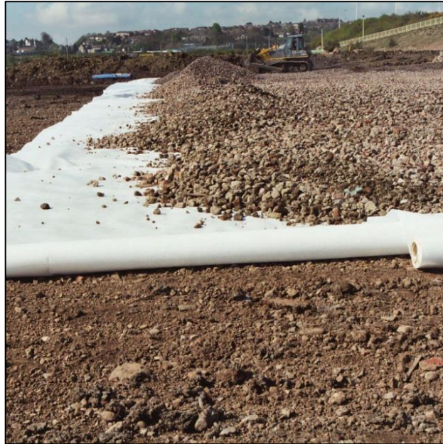
Figure 2.2 Geotextile reinforcement application.
