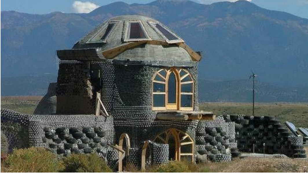
Görsel 5. Michael Reynolds, Earthship House (Çevre Dostu Ev). 2013. https://bit.ly/3exB1Qb
