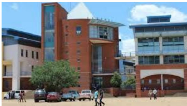
Figure 7. NUST Commerce building
