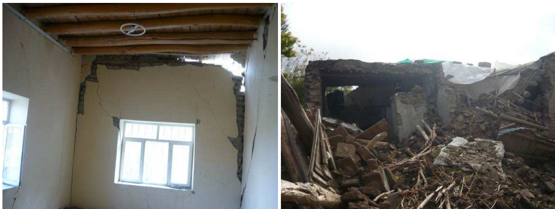
Figure 14. Flexible floor diaphragm
