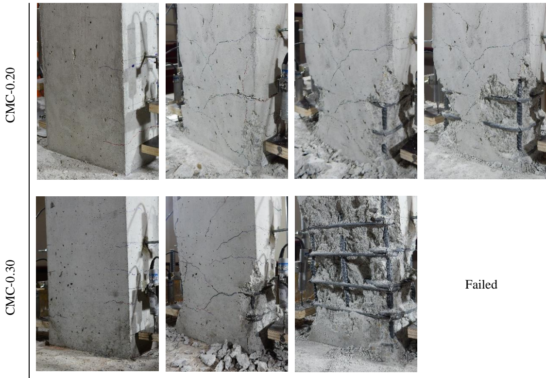
Figure 4.6 Damage progression in the monolithic specimens with increasing drift ratio
