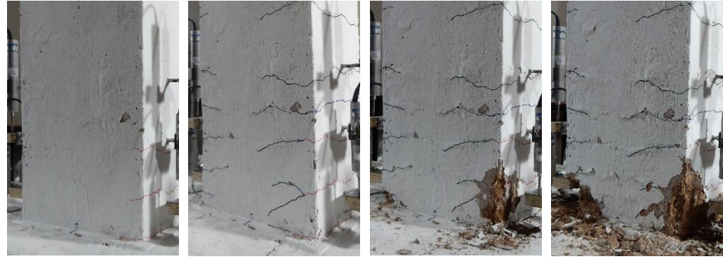
Figure 4.4 Observed failure modes at the monolithic specimens.
