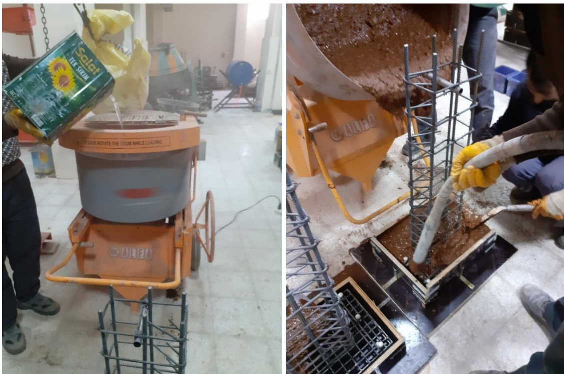
Figure 3.16 Preparation of the geopolymer mixture and casting into molds
