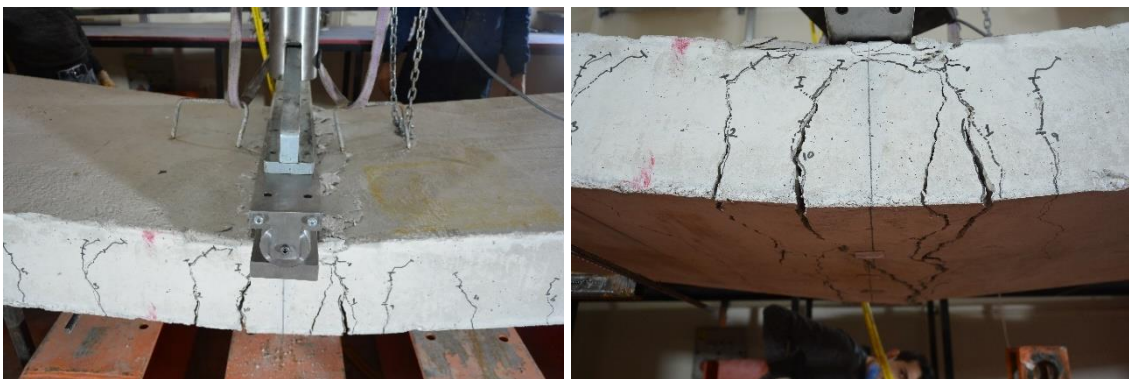
Figure 4.40 Failure of the demountable slab
