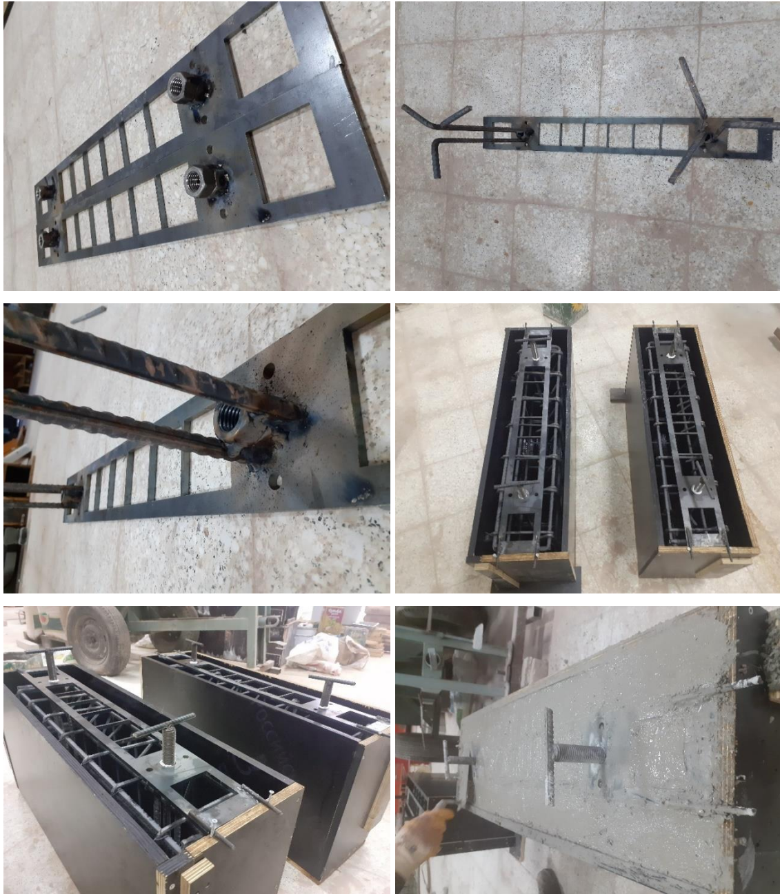
Figure 3.52 Structural details of beam body with pin-type slab connection via tie rods
