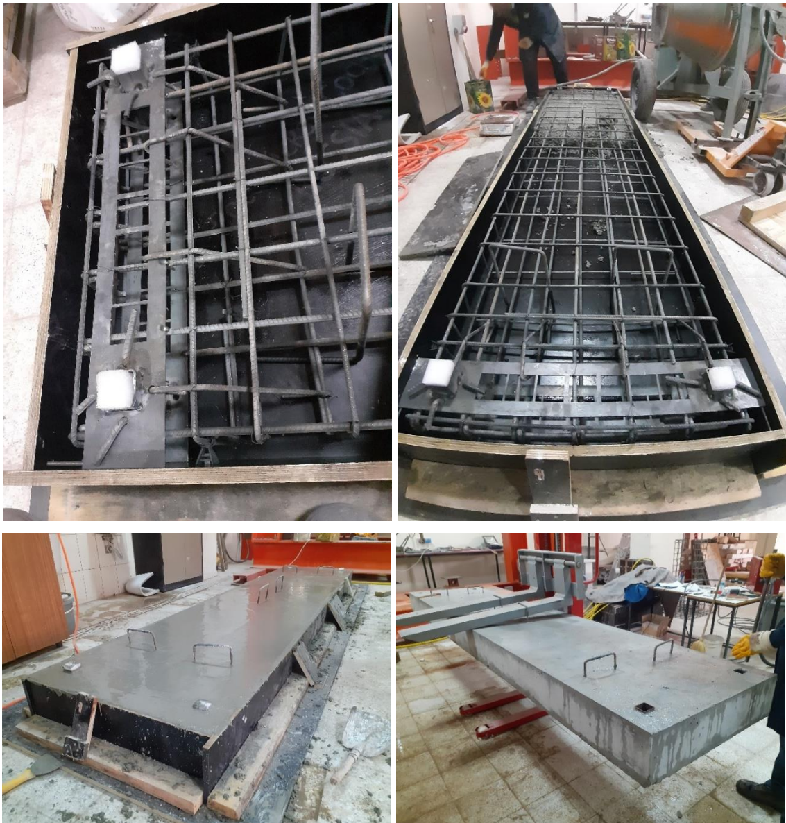
Figure 3.55 Details of demountable slab
