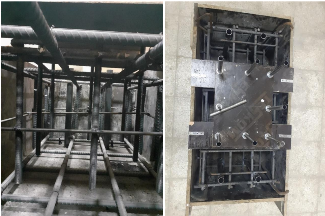
Figure 3.23 Vertical alignment of threaded rods
