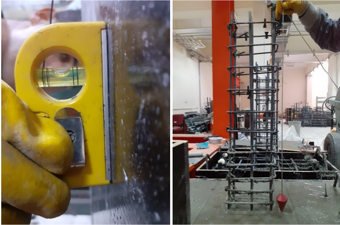
Figure 3.17 Preparation of the concrete mixture and adjusting the column plumb
