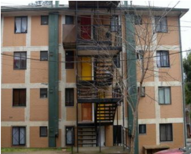
Figure 2.3. Confined masonry building
