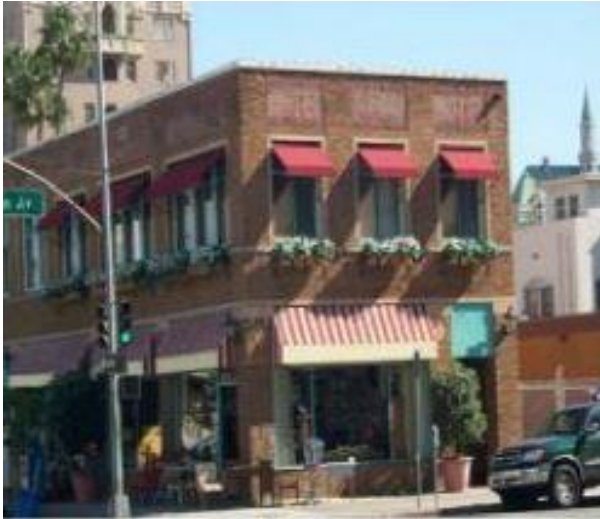
Figure 2.1. Photograph of an Unreinforced Masonry Building
