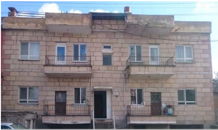
Figure 2.7. A building made of concrete block walls
