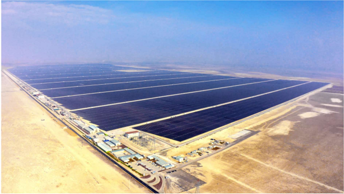
Figure 2.8 Konya Karapınar Solar PV Power Plant
