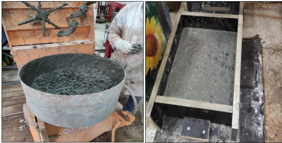
Figure 3.26. Substrate concrete casting
