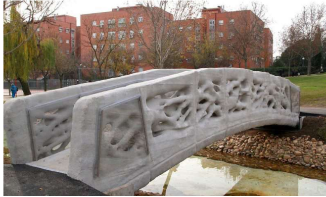
Figure 2.9 World's first 3D-printed pedestrian bridge [82]
