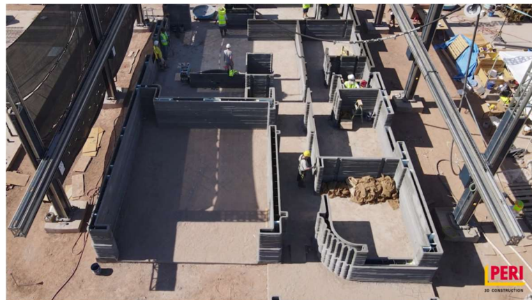
Figure 2.12 A bird's-eye view of the ongoing 3D printing of house [93]
