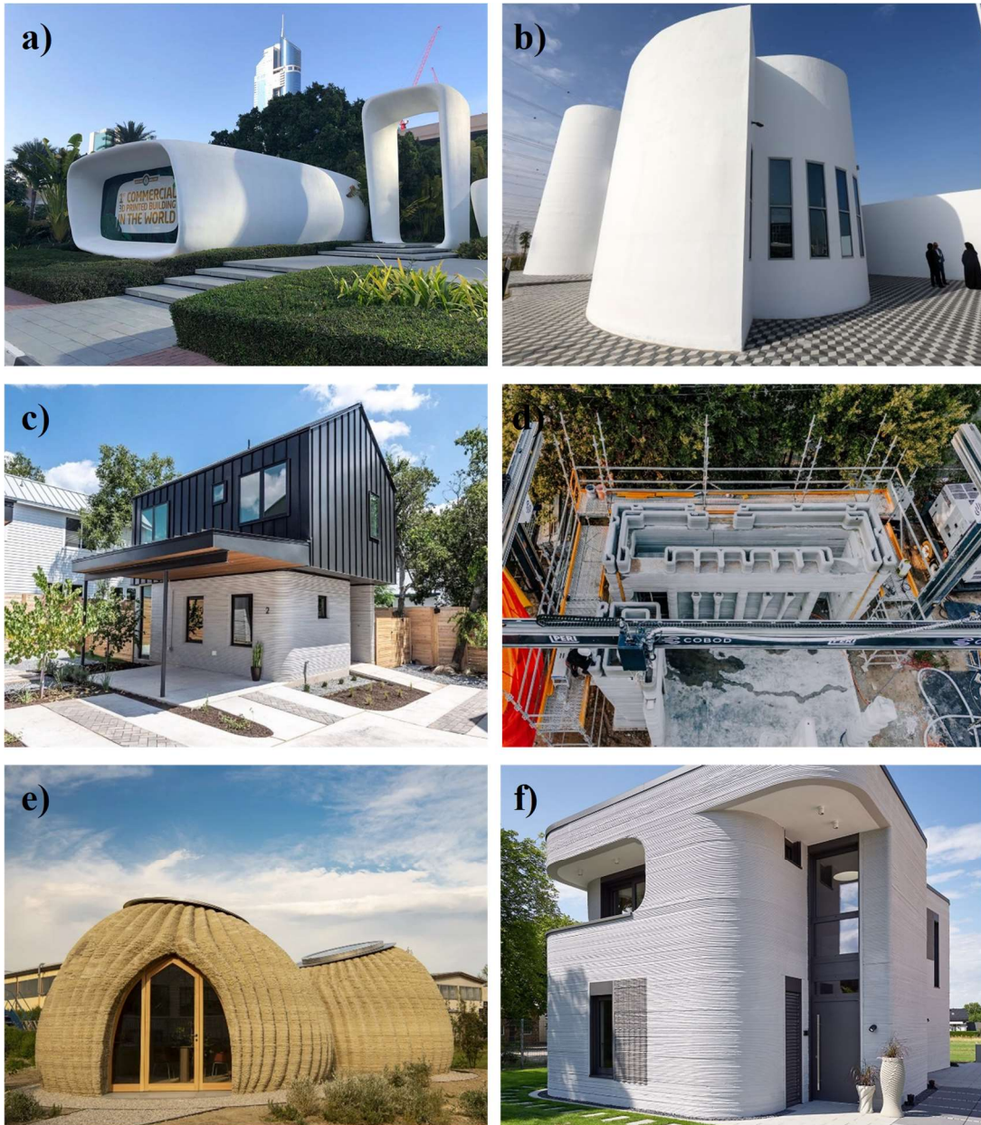
Figure 2.13 3D printed houses all around the world, a) Office of the future [96], b) World's largest 3D-printed building [97], c) Sustainable housing neighborhood [98], d) Two story 3D-printed house [99], e) Low carbon 3D housing [100], f) Two story 3D-printed family house [101]
