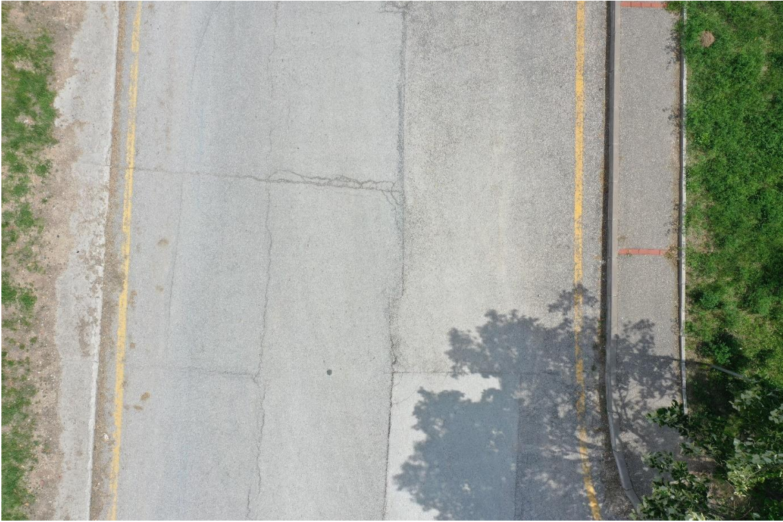
Figure 20. Example of road image collected using UAV
