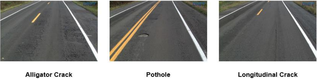
Figure 7. Samples of the images in the dataset introduced by Passos et al., (2020)
