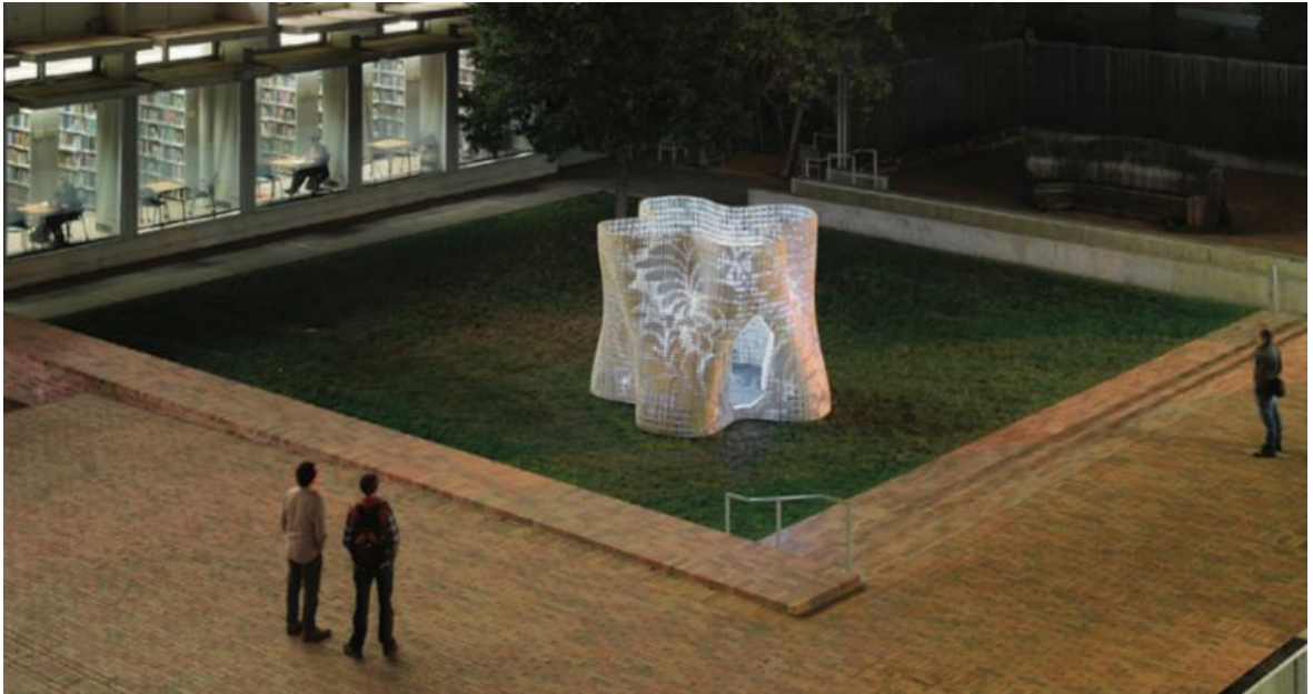
Figure 2.7 Bloom; an experimental pavilion that produced with 3D printed Portland cement [71]
