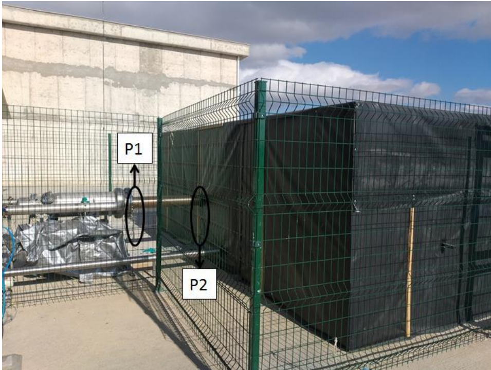
Figure 1-1. Free-Jet Nozzle Inlet Pressure Measurement Locations.
