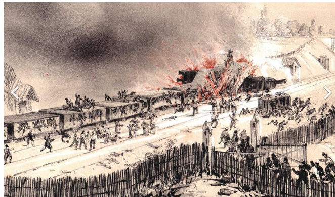
Figure 1.1 Versailles rail accident
