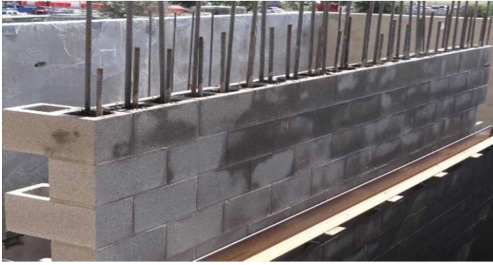
Figure 2.4. Reinforced Masonry Wall
