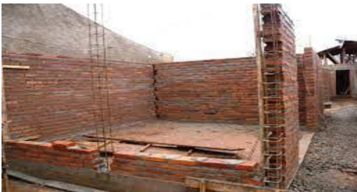
Figure 2.5. Confined Masonry Structures
