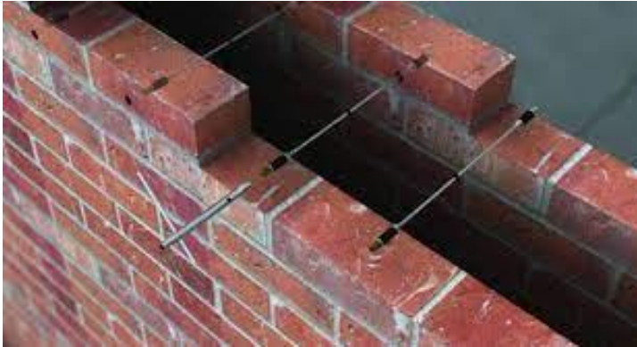
Figure 2.6. Cavity Wall
