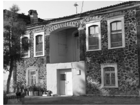
Figure 2. Cigerciler house, whole outside walls built with stones [12].
