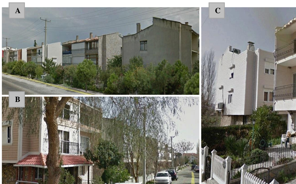
Figure 1.3. Three street level sample pictures regarding the study area taken from the Google Earth Images.
