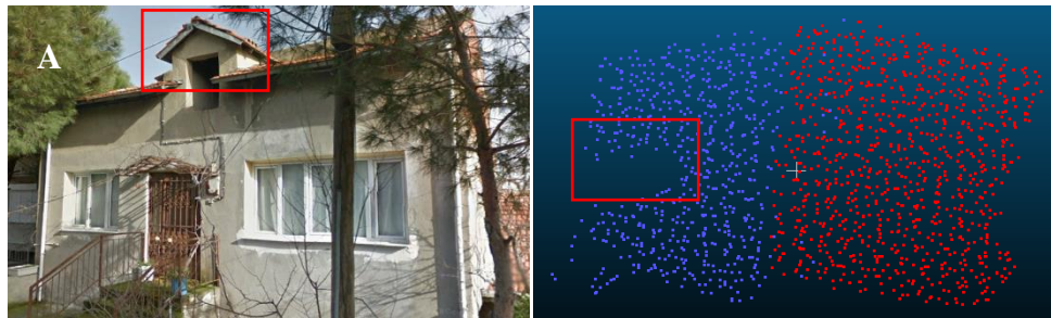
Figure 4.27. A. the building #28 with small window.
